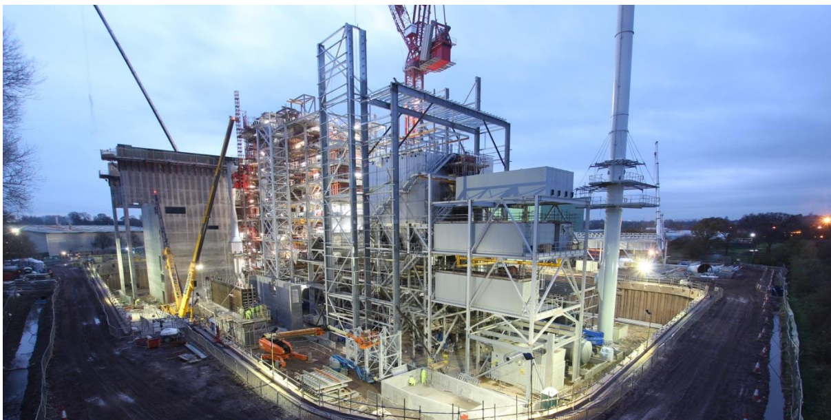
Envirecover Energy from Waste facility under construction.
